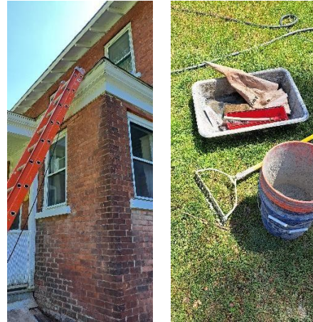
REPAIRED BRICKWORK AT THE PARSONAGE:
